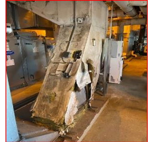
Inoperable HVAC Systems
