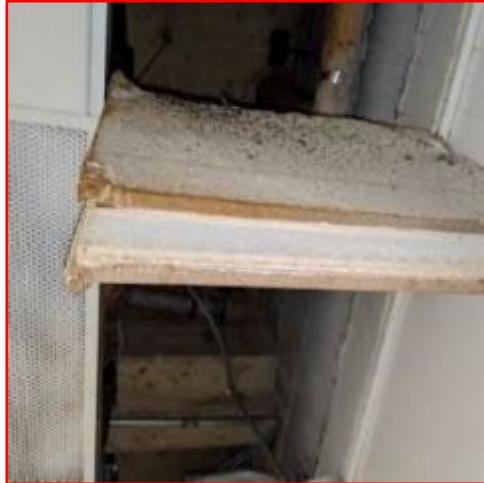
Black Mold Ceilings & Walls
