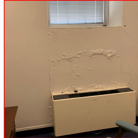
Water Damage & Infiltration
